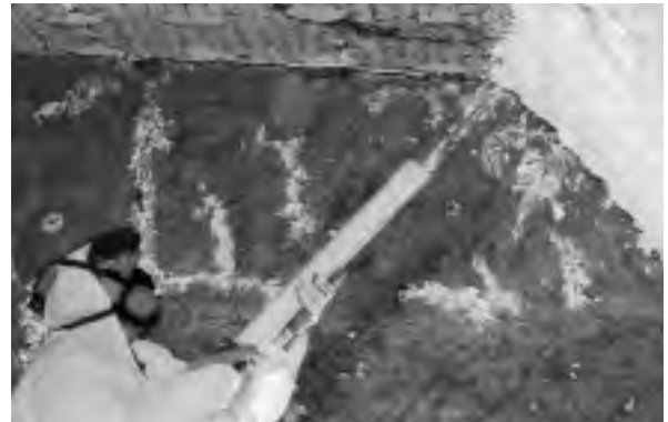
Projection d'Isofoam/Foamfrax
